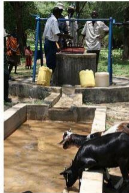
Figure 2: A well using a windlass and bucket to extract water for human and animal consumption. A dedicated livestock drinking trough separates the animals' water from the humans' water in Turkana, Kenya. Photo: Justine Williams / Practical Action
