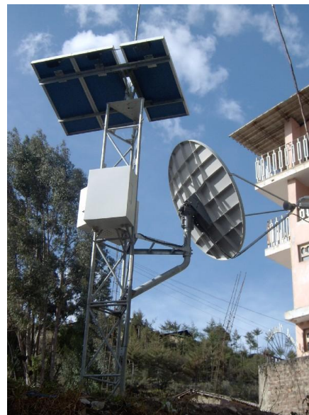
Figure 3: The La Encanada infocentre, Peru has solar panels to generate electricity and a satellite for connectivity. Photo: Practical Action / Jaime Soto.
