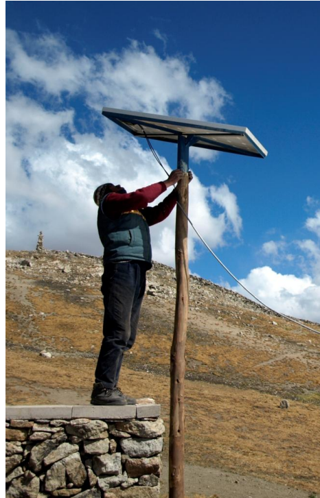
Figure 1: A photovoltaic panel being set up in rural Peru for domestic solar lighting. Photo credit: Practical Action / Marco Antonio Arango.
