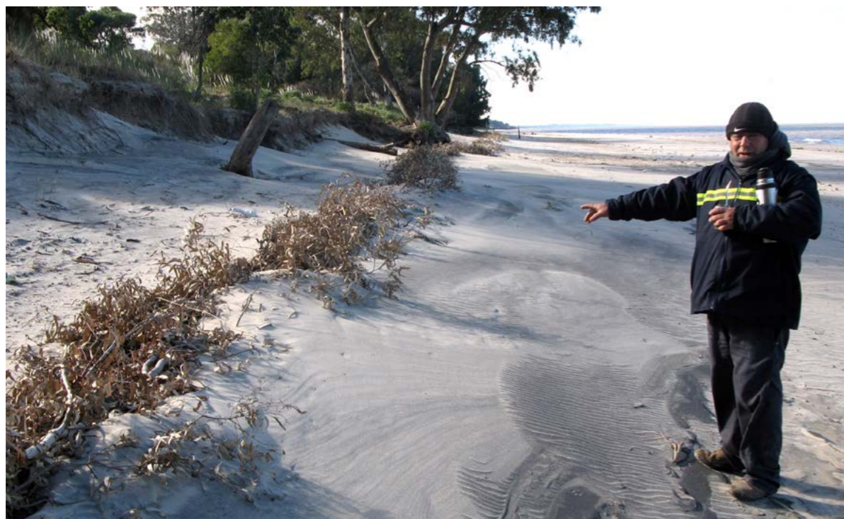
Photo: Intermediate results of sand accumulation in capturing fences. Project archive
