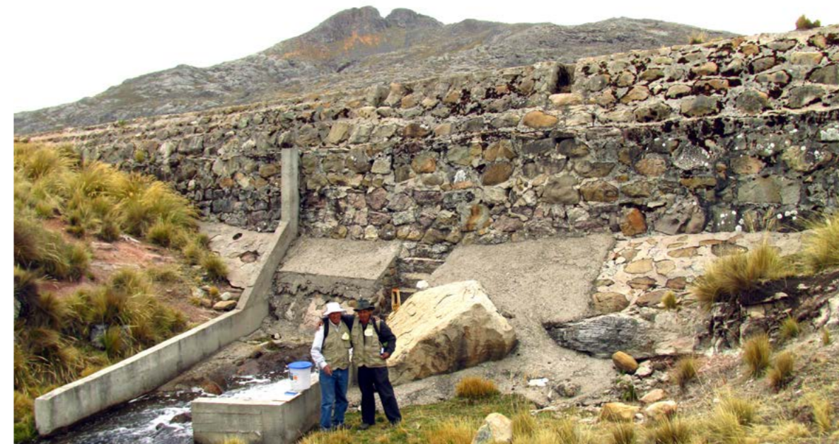
Photo: Infrastructure improvement in Canchayllo. Project archive
