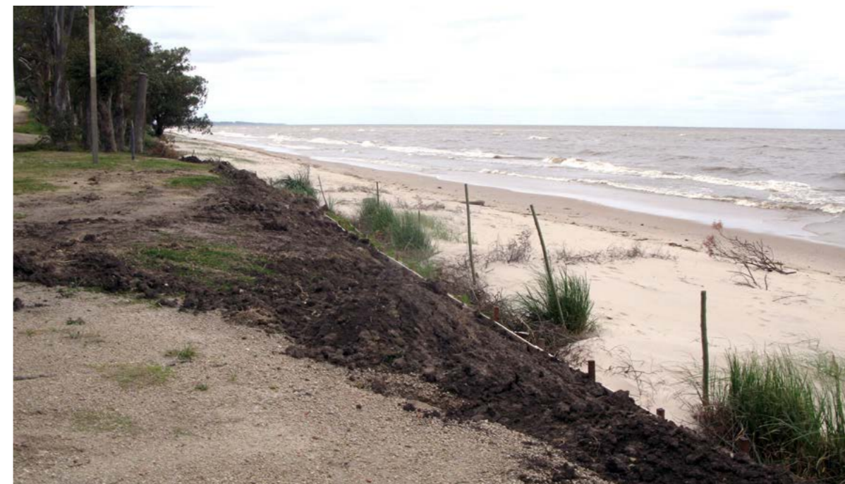
Photo: Works of reprofiling canyons. Rain damping. Project archive
