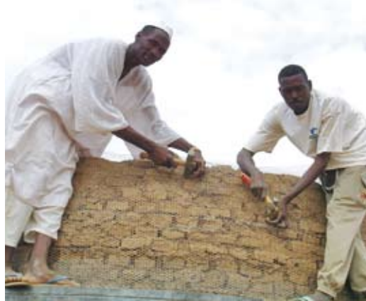
Pic 16. The wire mesh is tied around the partly made dome
