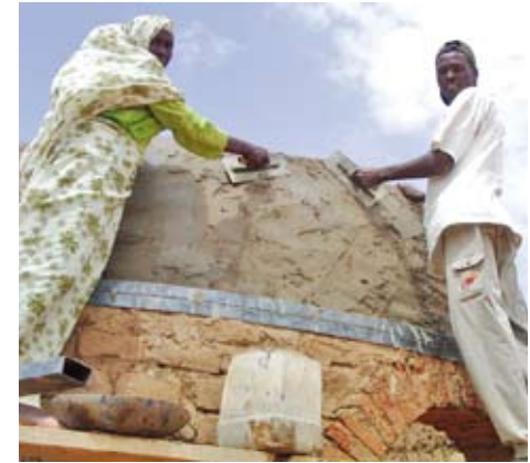
Pic 17. Cement is plastered on top of the wire mesh
