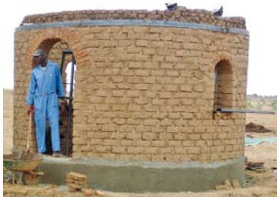
Pic 14. Bricks are laid for the formation of the dome
