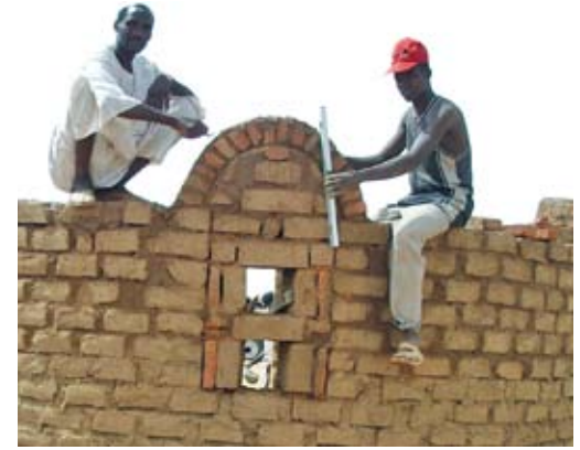
Pic 10. The window arch using method 2
