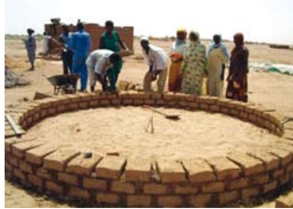
Pic 6. The wall reaches three courses in height
