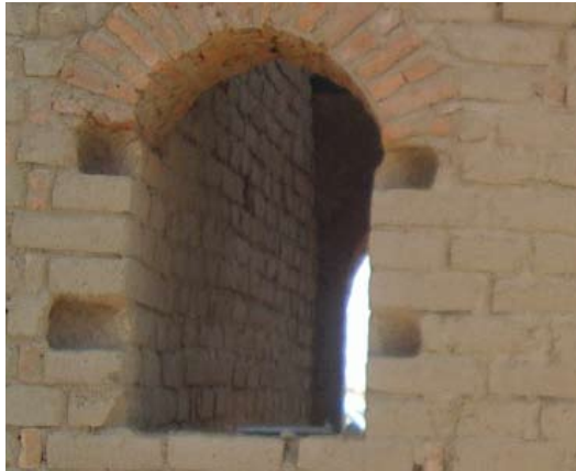
Pic 25. Four holes are made around the sides of the window hole
