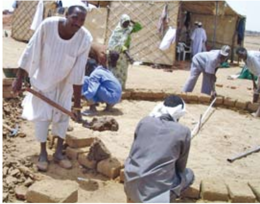
Pic 5. The tape and peg are used for marking the radius of walls
