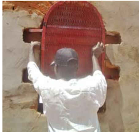
Pic 26. The window frame is inserted
