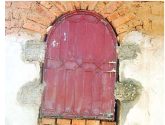
Pic 27. Cement is used to fix the window frame in place
