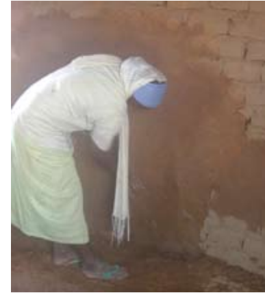
Pic 24. A lady plasters the inside walls
