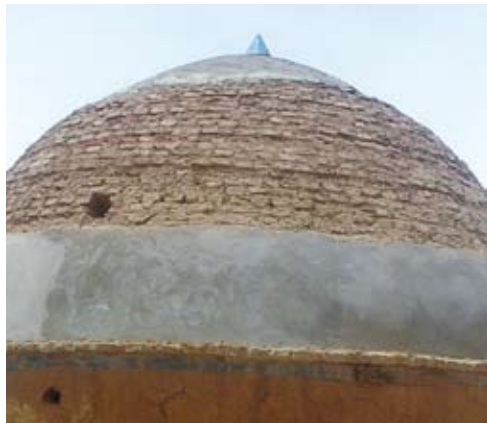
Pic 21. The metal hole cover can just be seen at the top of the house
