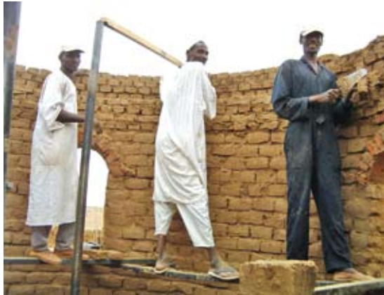
Pic 15. The dome measuring tool is used to form the dome.
