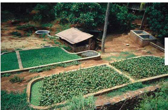
Figure 4: Sewage system using water hyacinth. ©Paul Calvert/Practical Action
