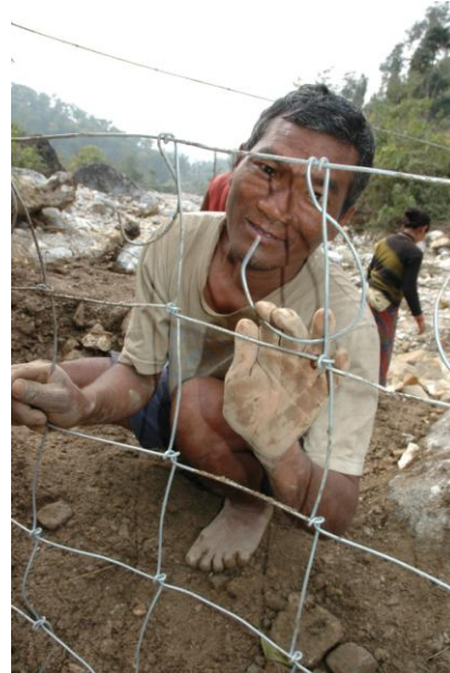
Figure 5: Making gabion cages by hand with a square mesh. Photo: Practical Action Nepal
