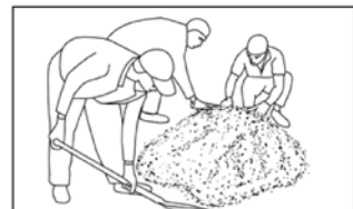
Mix 2 nd time & crush lumps by hand
