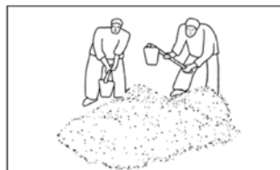
Always move the pile while mixing
