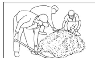
Mix 2 nd time & crush lumps by hand
