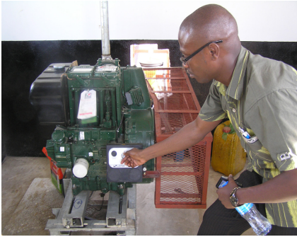
(a) Diesel engine (left) supplying power to a borehole pump via a belt drive (right, in cage), Tanzania
