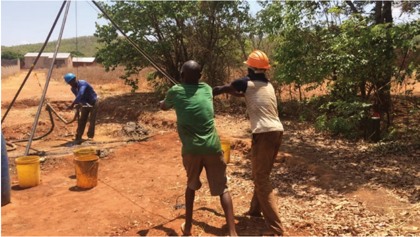
Photo CS.5.1 SHIPO hand-drilling
