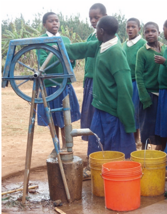
Photo CS.5.2 Contractors sell low cost options for community projects as well as self-supply, this school supply was installed 15 years ago
