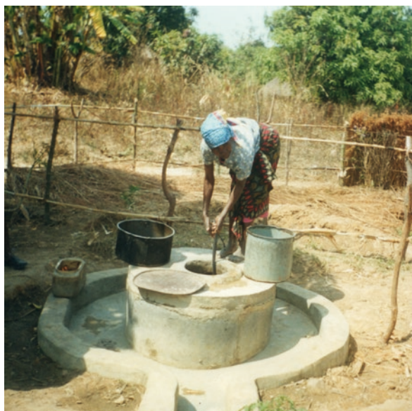
Photo 7.5 The well in Photo 7.2 with basic improvements including a pole for hanging up the rope and bucket
