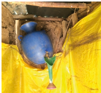
Photo 6.16 Homemade shower using storage pot and watering can rose, Ethiopia
