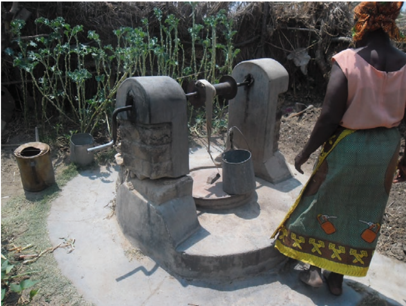
Photo CS.4.2 Family well showing a lack of attention and maintenance
