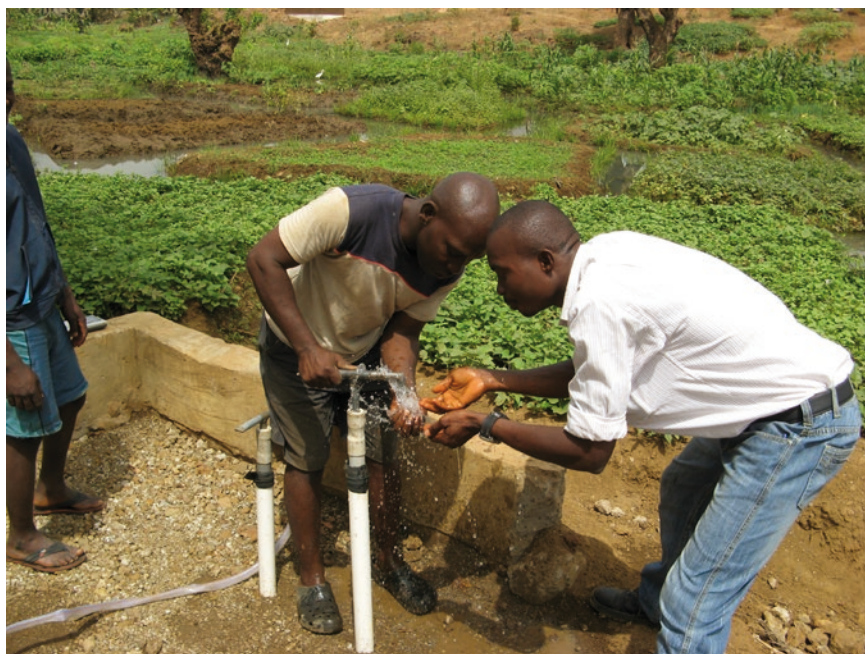
Photo 6.13 EMAS pumps for demonstration in Sierra Leone
