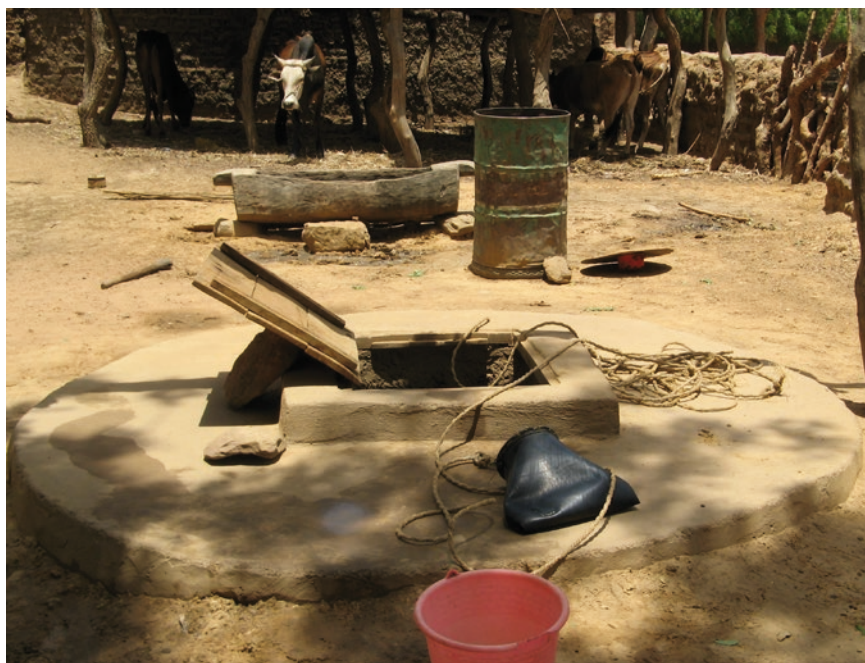
Photo 5.2 Household well with cattle trough and cow-shed; domestic and productive uses from on-premises self-supply well, Mali
