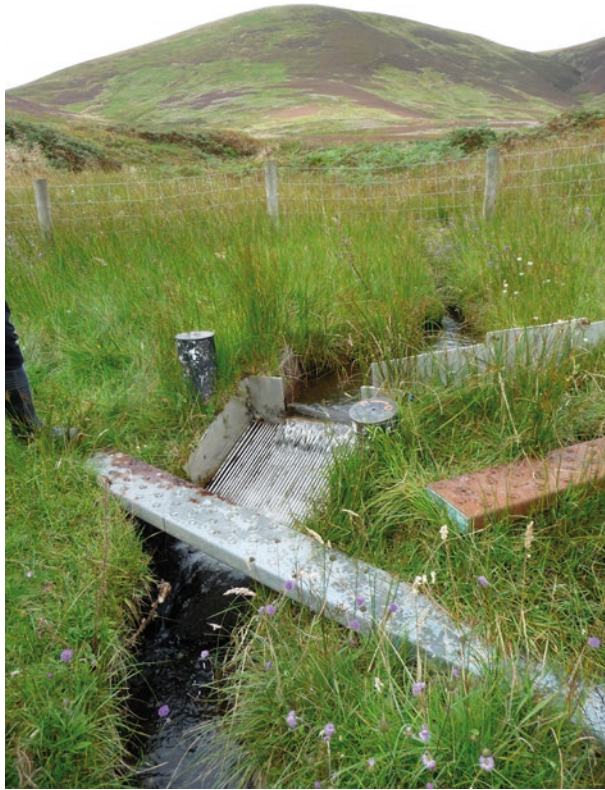
Photo CS.1.1 A reasonably well-designed and maintained private surface water abstraction in rural Scotland, with a 'stilling pool' upstream and a screen to remove coarse debris Source: DWQR
