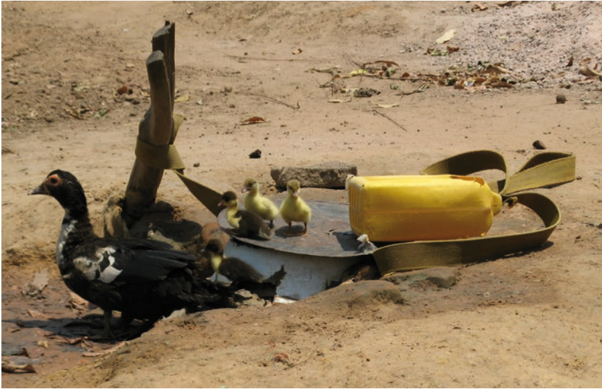
Photo 7.2 Unimproved wellhead, Luapula province, Zambia
