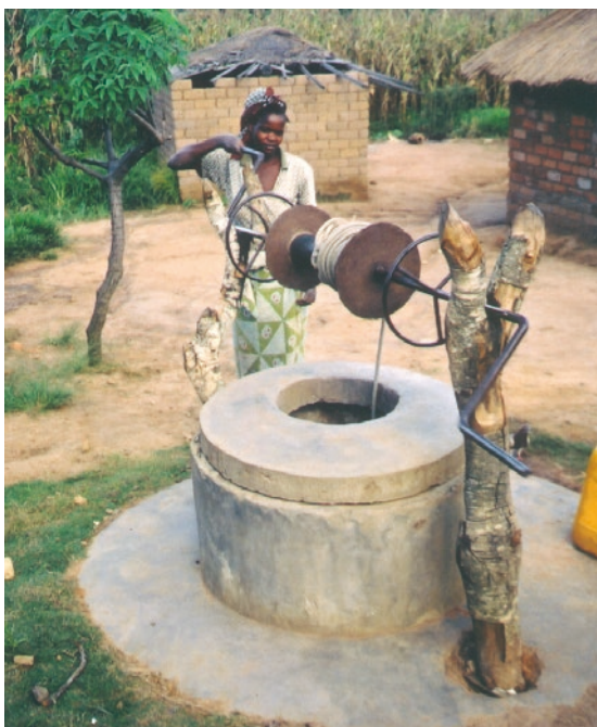
Photo 7.4 The well in photo 7.1 improved by the household, but still lacking a cover or drainage
