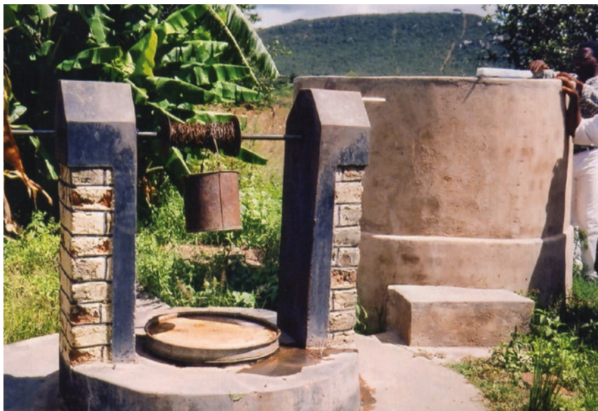
Photo 3.1 Upgraded Zimbabwean family well with cistern for small-scale irrigation
