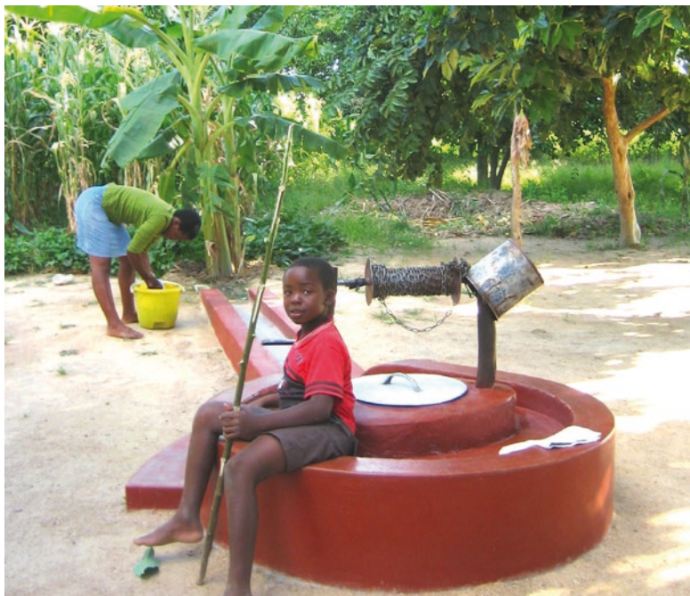
Photo CS.4.1 Well built during Zimbabwe's National Upgraded Well Programme
