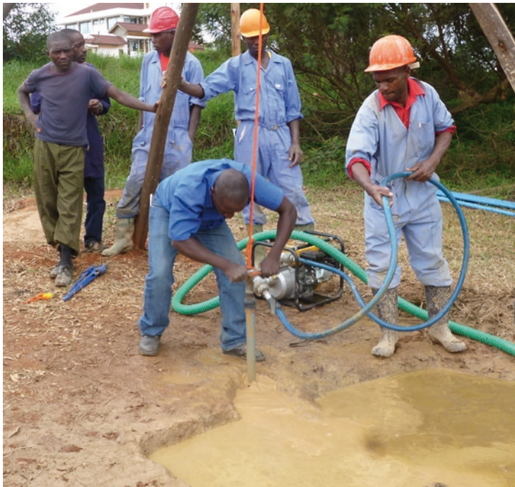
Photo 6.8 SHIPO drilling in Tanzania Source: Photo H. Holtslag
