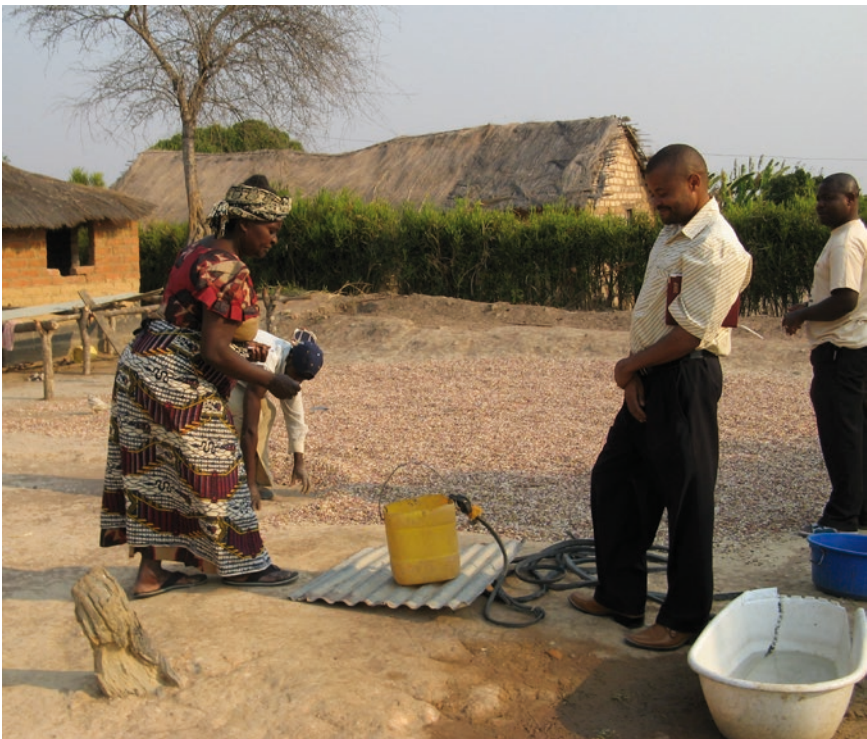
Photo 7.3 Household well covered but with no other protection, Luapula Province, Zambia
