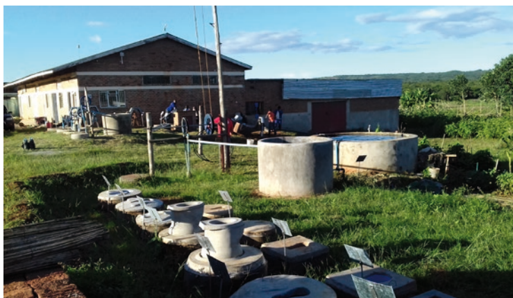
Photo 6.21 SMART Centre in Mzuzu, Malawi
