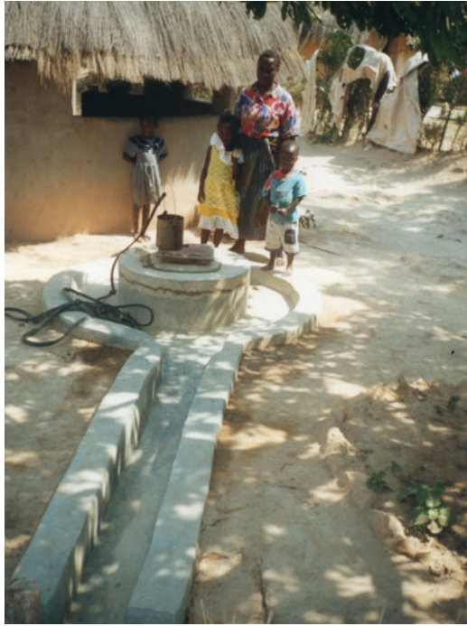
Photo 7.6 The well in Photo 7.3 with basic improvements including lockable cover
