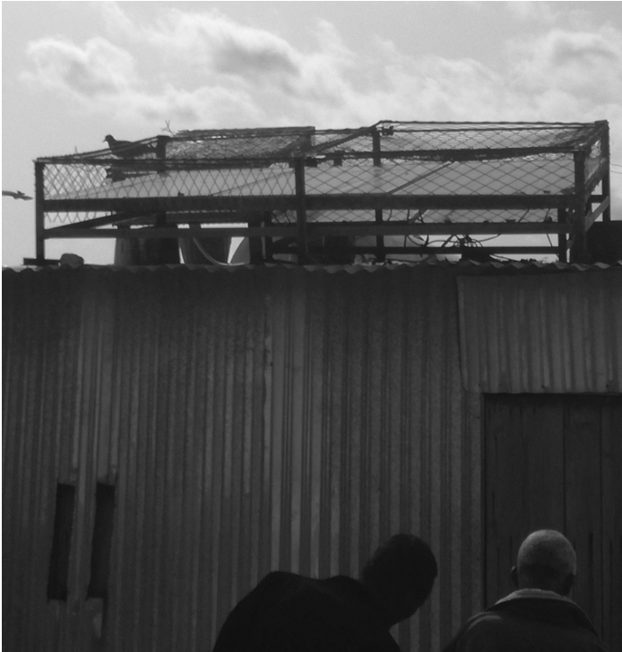
Figure 7.4 Extreme module security measures in Burao, Somalia
