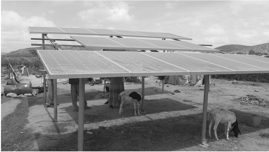
Figure 4.4 Sand on PV modules limiting power output
