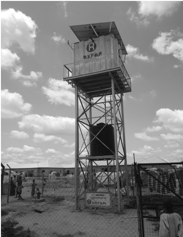
Figure 6.13 Tank-mounted structure in an IDP camp near Maiduguri, Nigeria
