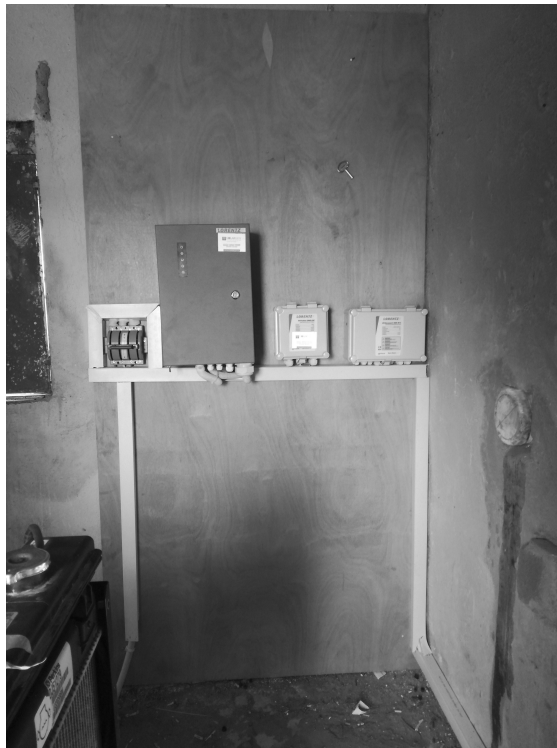
Figure 6.4 Installed controls (left to right): AC changeover switch, inverter, surge protector, PV disconnection switch
