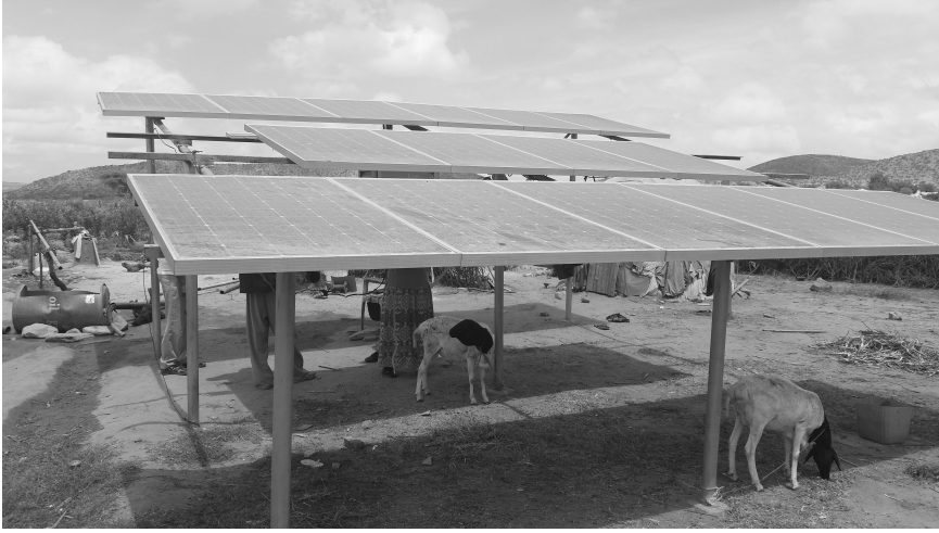
Figure 4.4 Sand on PV modules limiting power output
