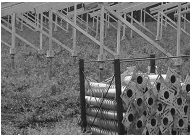
Figure 6.12 Example of ground screw structure
