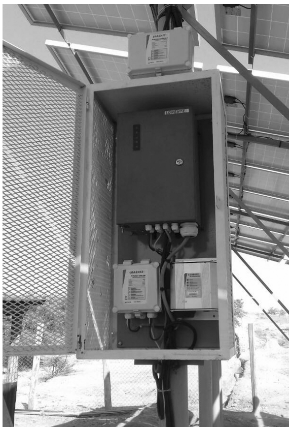
Figure 6.5 Inverter installed in a lockable meshed enclosure under the PV array at Turkana, Kenya Source: Oxfam
