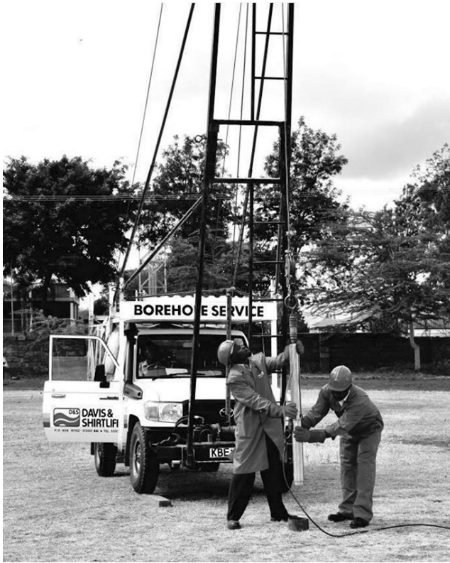
Figure 6.2 Pump installation using a hydraulic winch
