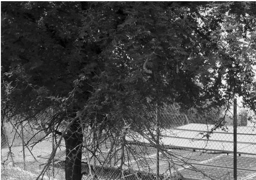
Figure 4.5 Shading of PV modules limiting power output
