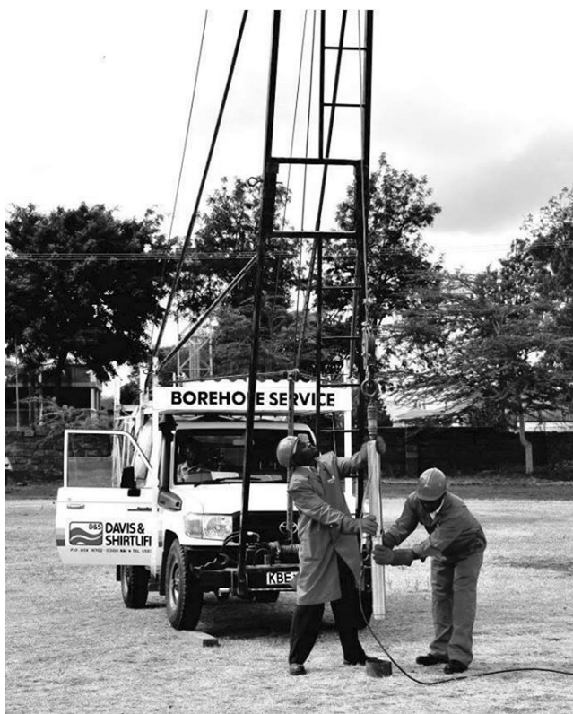
Figure 6.2 Pump installation using a hydraulic winch
