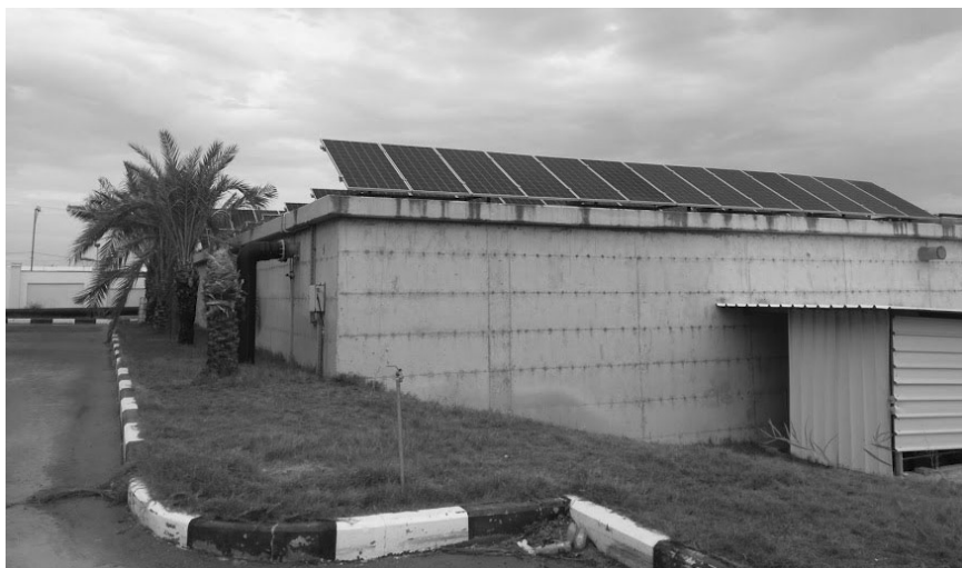
Figure 6.10 Roof mount on a flat tank roof in Gaza
