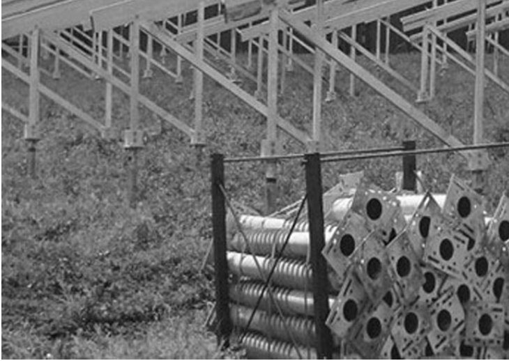
Figure 6.12 Example of ground screw structure
