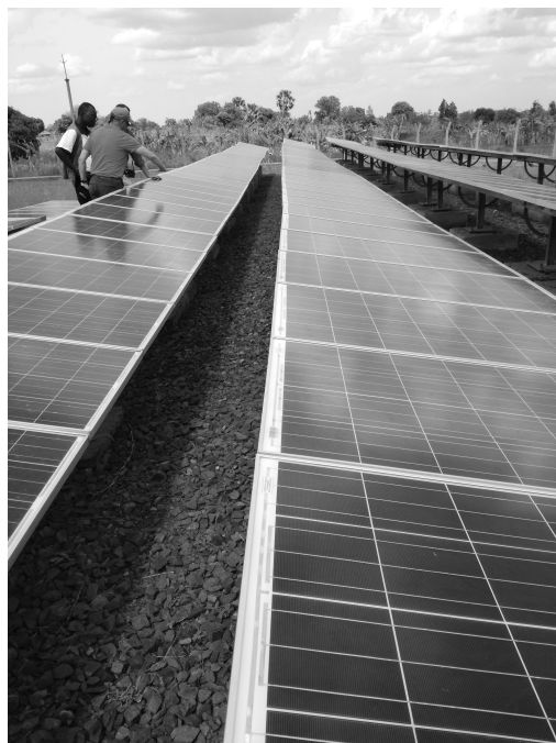
Figure 6.19 Walkway on a ground mount in Koboko, Uganda
