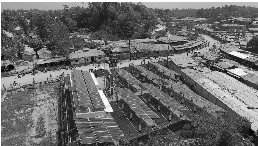
Figure 6.11 Combined roof and pole mount installation at IOM water scheme, Kutupalong Balukhali Expansion Site refugee camp (Cover photo)
