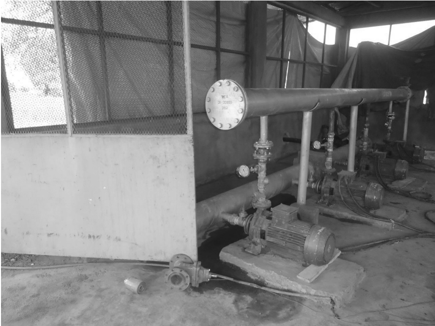
Figure 6.3 Horizontal surface pumps installed on a concrete plinth in Itang Water Supply, Ethiopia
