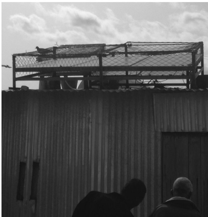
Figure 7.4 Extreme module security measures in Burao, Somalia
