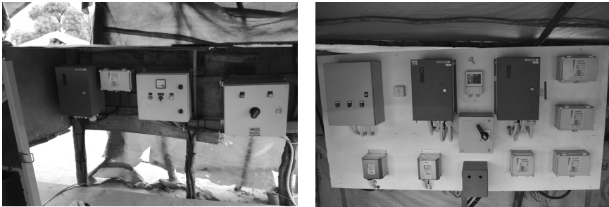
Figure 6.7 Examples of good cable management in South Sudan and Tanzania respectively
