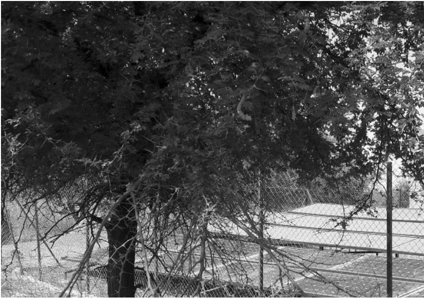
Figure 4.5 Shading of PV modules limiting power output
