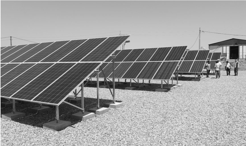
Figure 5.7 PV modules in Sheikhan, Iraq, facing south at 36^\circ tilt
