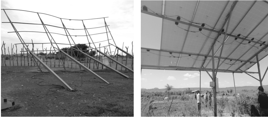
Figure 6.14 Failed pole mount in Yida, South Sudan (left), modules blown off in Fafen, Ethiopia (right)
