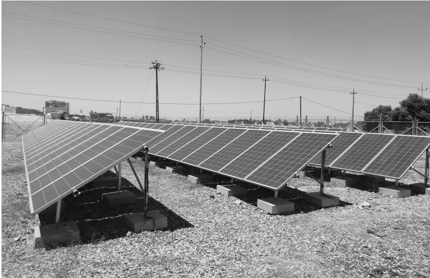
Figure 6.8 Ground mount structure in Kawrgosk refugee camp, Iraq
