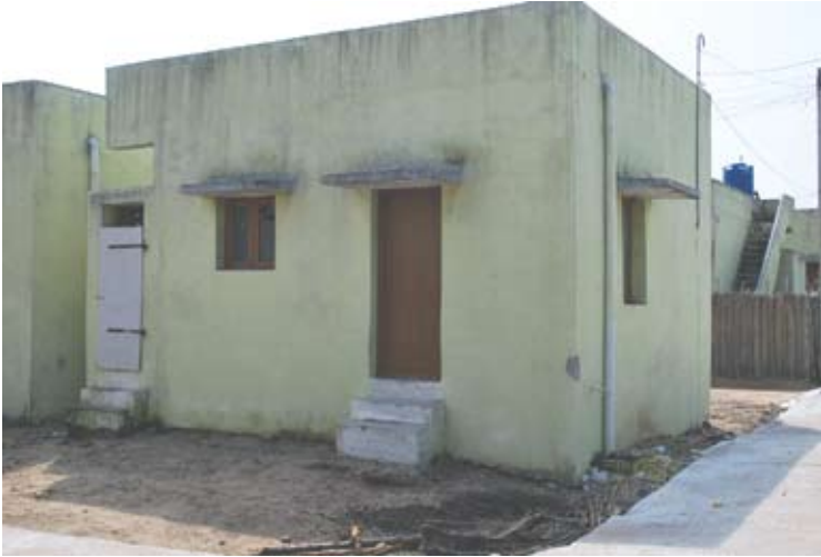
Figure 3.11 Example of house built by one of the agencies involved in the reconstruction of Seruthur
