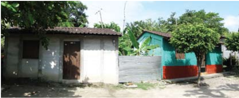
Figure 12.5 Concrete panel houses in the Edin Martinez community: house on the left – no changes made since its handover; house on the right – painted façade, doors and floor changed
