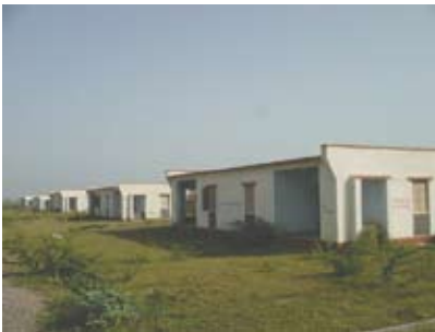
Figure 3.8 Empty agency-built houses in Fadsar in 2004
