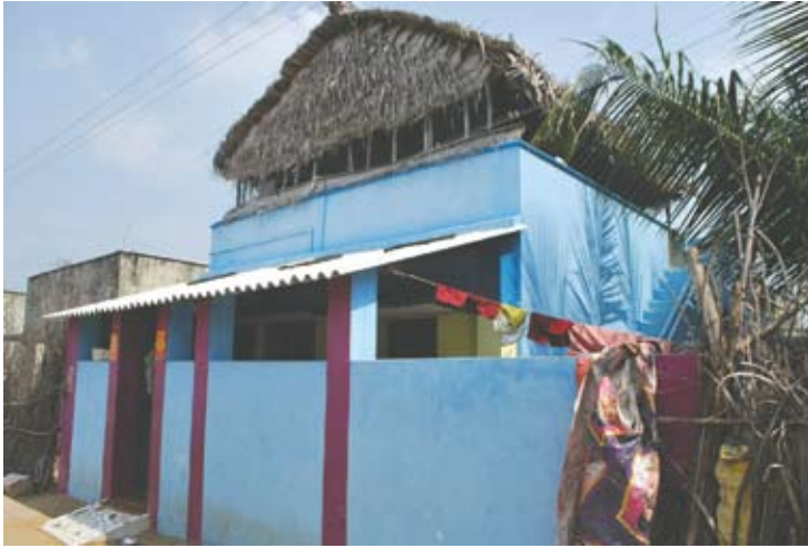
Figure 3.12 Example of extensions of an agency-built house in Seruthur
