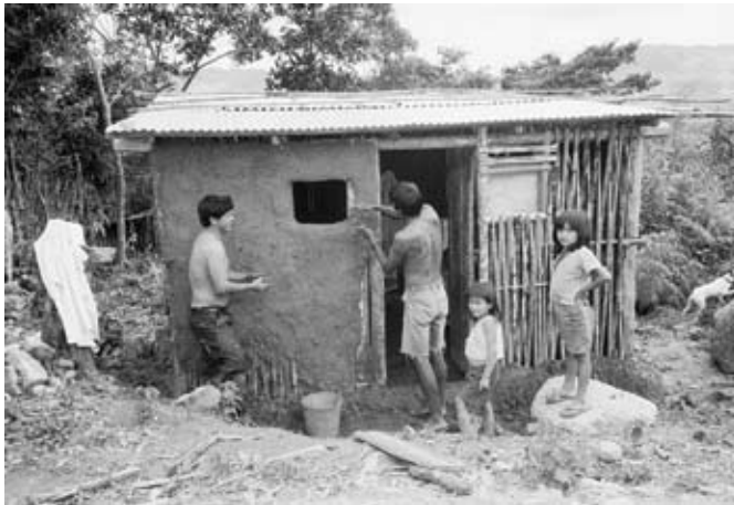
Figure 13.2 Traditional quincha house under construction in the Alto Mayo of Peru
