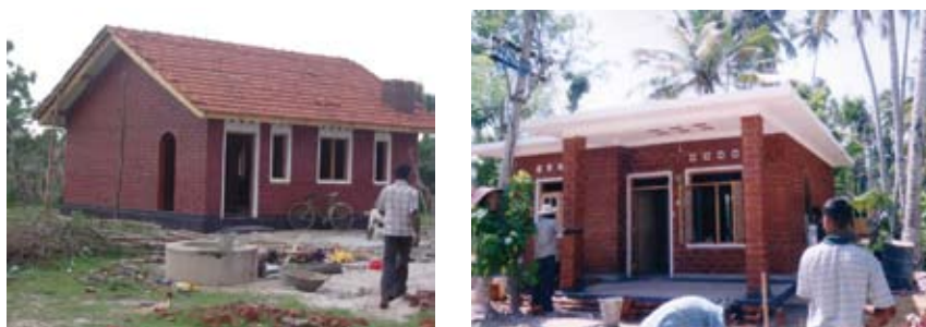
Figure 6.2 and 6.3 Rat-trap technology topped with a tile roof (house on the left) and a flat roof showing ventilation holes in white below (house on the right)
