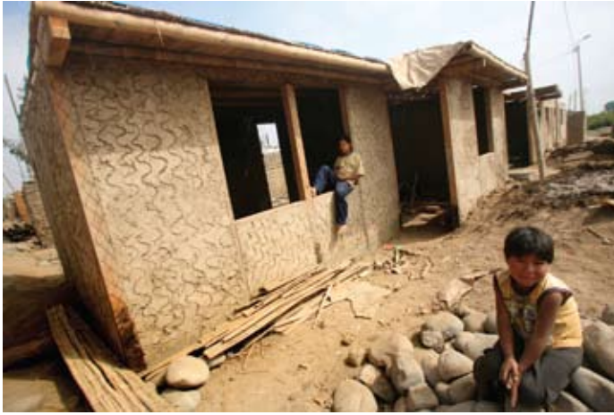
Figure 13.4 Improved quincha houses during construction
