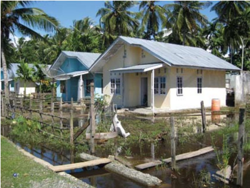
Figure 2.1 Flooded houses in Indonesia at the time of the assessment
