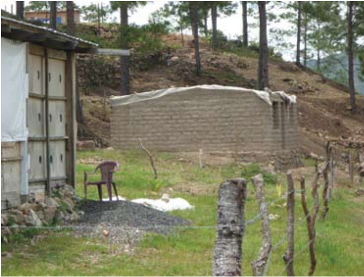
Figure 10.5 Illegal but apparently tolerated, 'soft invasion' with low-cost housing
