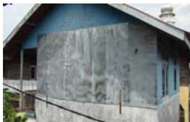
Figure 8.6 Wooden wall covered with metal sheeting to protect it from rainwater
