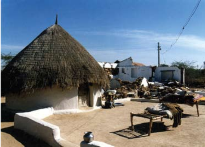
Figure 5.2 After the earthquake, Ludiya, 2001
