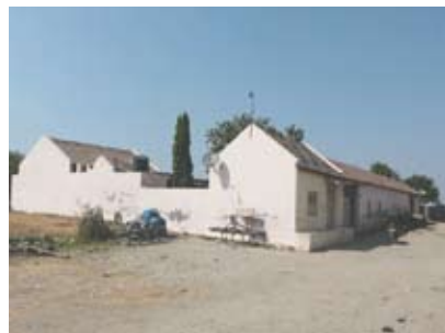
Figure 3.9 A transformed large house in Fadsar in 2012
