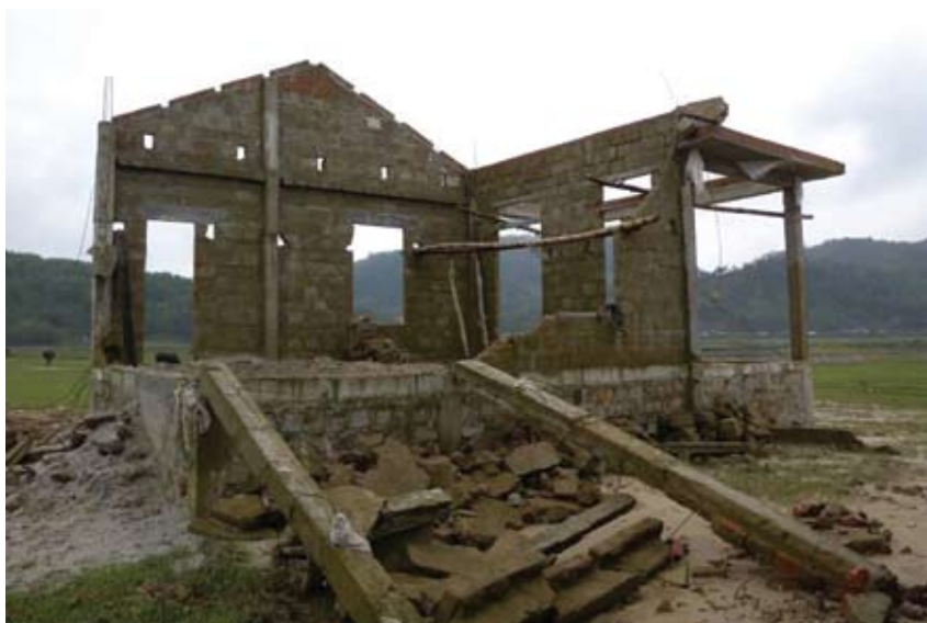
Figure 7.3 Dwelling under concrete plinth, reinforced concrete frame and cement block retaining wall, with the interior filled with sand up to the raised floor level
