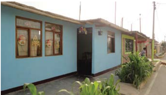
Figure 13.7 Several houses in a row that have been well finished, the farthest with 'imitation-brick' paint and metal windows
