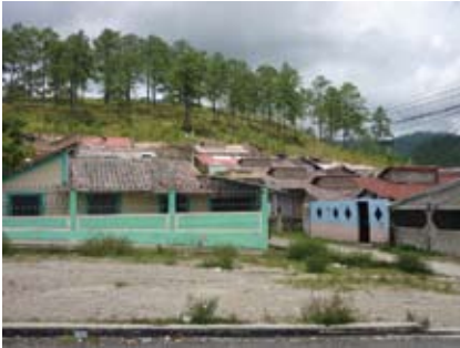
Figure 10.6 People have made additions but the architectural unity is preserved
