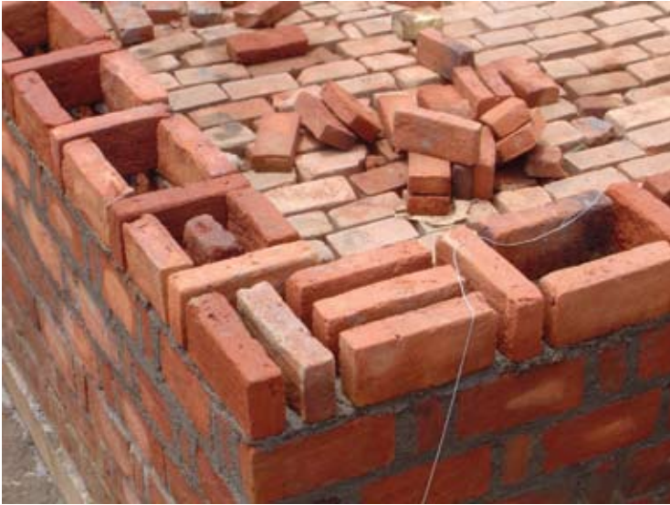
Figure 6.1 Rat-trap technology, used in India and introduced by Practical Action post-tsunami after an earlier trial in north-western Sri Lanka
