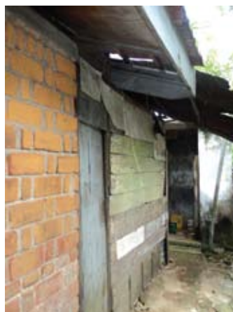
Figure 6.5 Galle house with boarded extension
