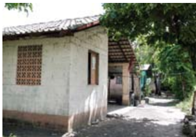
Figure 11.7 Houses are in good repair
