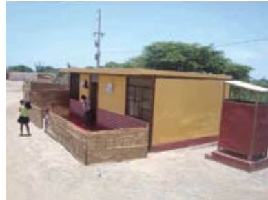
Figure 13.6 Painted improved quincha house, including an 'imitation-brick' lower part
