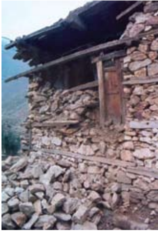
Figure 4.4 Traditional building with wooden tie beams
