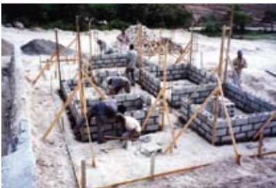
Figure 10.1 Guided self-help construction
