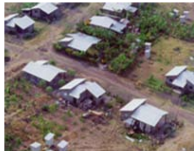
Figure 11.2 Aerial view of the houses showing the variety of design
