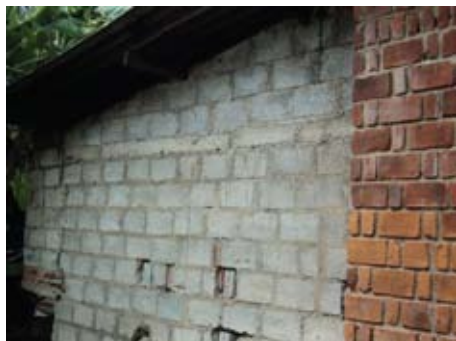
Figure 6.4 Galle house extension constructed with concrete blocks
