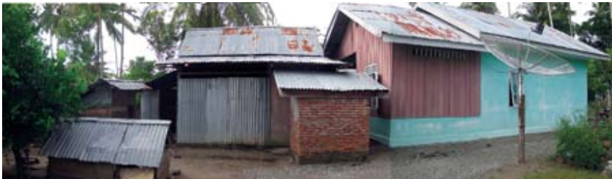
Figure 2.3 HFH's core home design (far right) in one community in Indonesia which incorporates the re-use of a timber transitional shelter as a kitchen (right) and later extensions using a combination of timber and other materials (centre and left)
