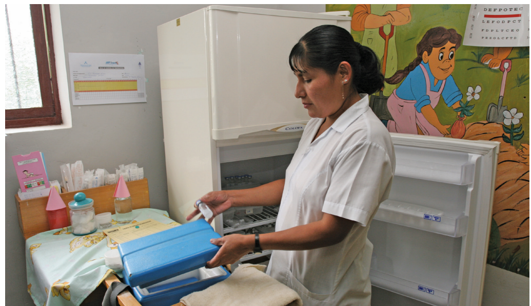
Refrigeration keeps vaccines cool at the health centre in Tamborapa, Peru. Power is supplied to this remote community via a micro-hydro system (Practical Action)
