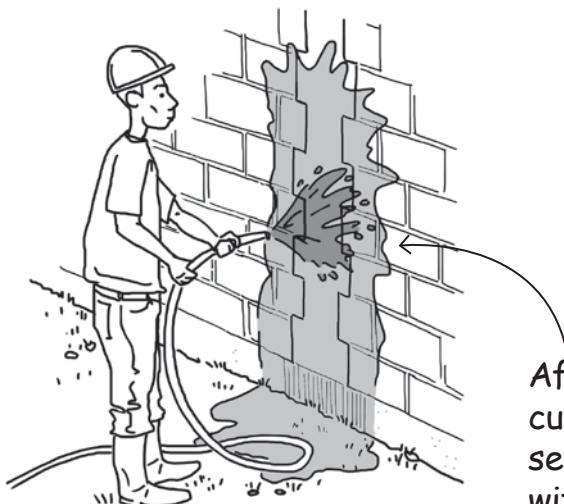
After formwork is removed, cure the concrete for seven days, and cover it with plastic sheets.
