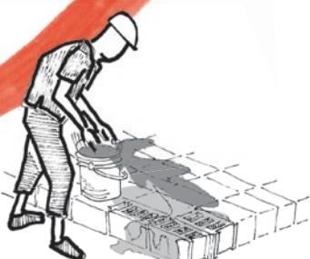
Cure the blocks three times a day for **minimum seven days** and cover with plastic sheets.
