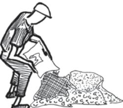
1. Make a pile with the gravel, the sand and the cement but without water.
