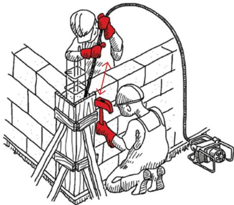
Pour the concrete in layers of 30 to 60 cm and compact well with a rod and hammer, or better, with a vibrating needle.
