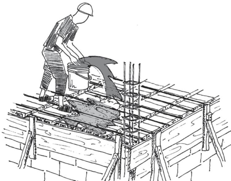
Water the formwork before pouring the concrete.
