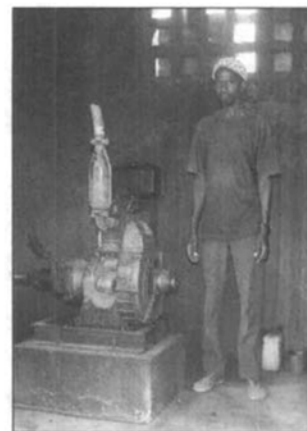
The mechanic and the 1hp pump motor for the borehole at Diass.
