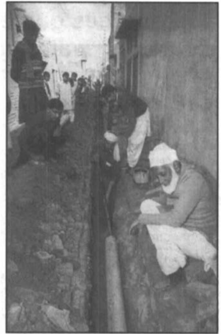
Community-laid pipes (that work!)
