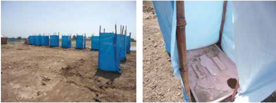
Newly built latrines in a small IDP camp near Jacobabad, Pakistan 2010. There is little privacy, no cleaning organized and as a result they were not used. Thousands of these types of latrines were built in the Sindh and Baluchistan provinces after the flooding disaster. Photos: Rink de Lange
