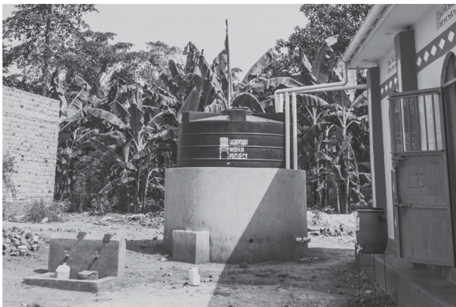
Photo 1 Photograph of a completed RWH system installed by the Ugandan Water Project
