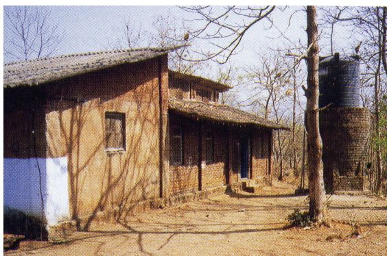
Figure 3 High-level water tank for treatment by sedimentation
