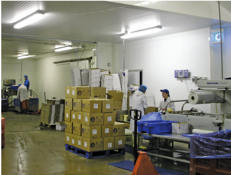
Figure 2 Hygienic PVC wall and ceiling panels Source: Courtesy of Hygienic (Clad & Clean) Ltd
