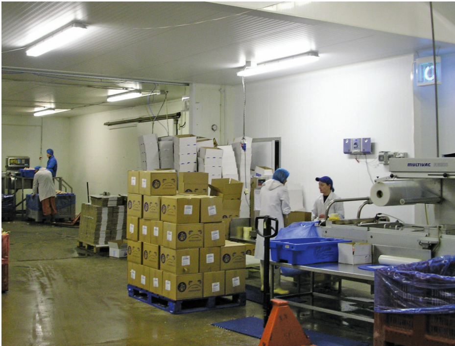
Figure 2 Hygienic PVC wall and ceiling panels Source: Courtesy of Hygenic (Clad & Clean) Ltd
