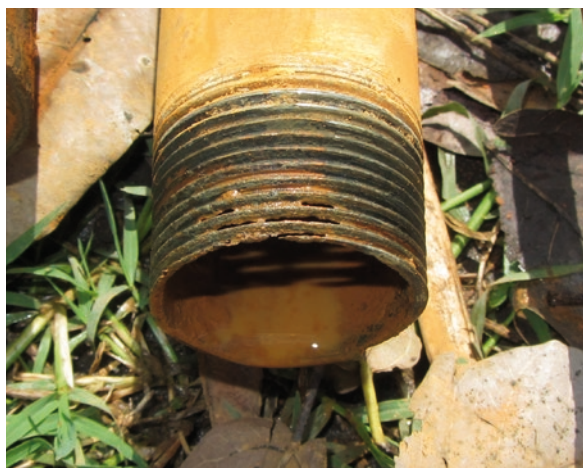
Figure 6 Threads on riser pipe at Odengelo, one year after installation
