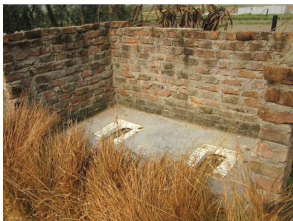
Photo 3 Subsidies remove the incentive for households to invest their own funds in a toilet and appear to change the way people think about toilets. Above, a subsidized double toilet with a half-completed superstructure. The household was waiting for an additional subsidy to finish the toilet.
