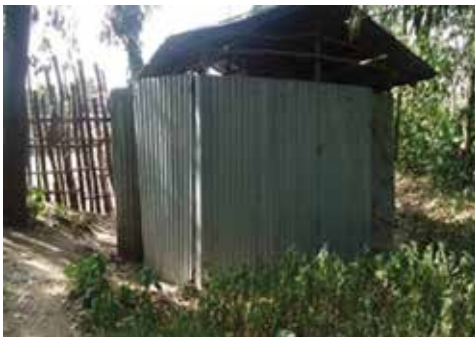
Figure 2 Toilet facilities for girls at Enseno Secondary School, Meskan district, Ethiopia (exterior)
