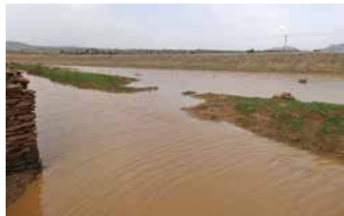
Figure 1 Waterlogging behind a road embankment along the Freweign-Hawzien road, Northern Ethiopia
