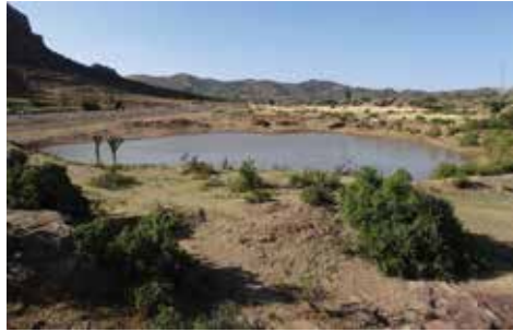
Figure 2 Pond used to harvest runoff from culverts for livestock and groundwater recharge in Wukro area, Tigray, northern Ethiopia Credit: photo by Kifle Woldearegay, July 2013
