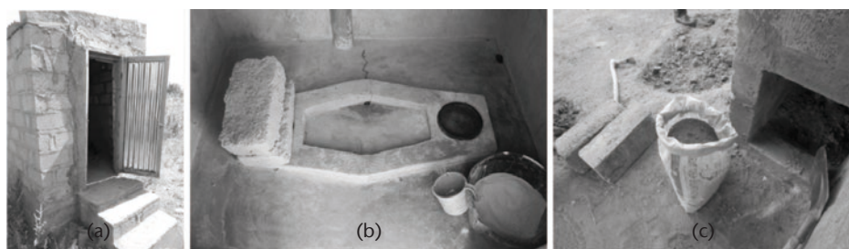
Photo 1 The common double vault UDDT in Burkina Faso. The urine diverter is often cast in cement on the slab, and there is an outlet for anal wash water in the corner of the cabin (b). The vaults can be emptied, removing the cover bricks (c).
