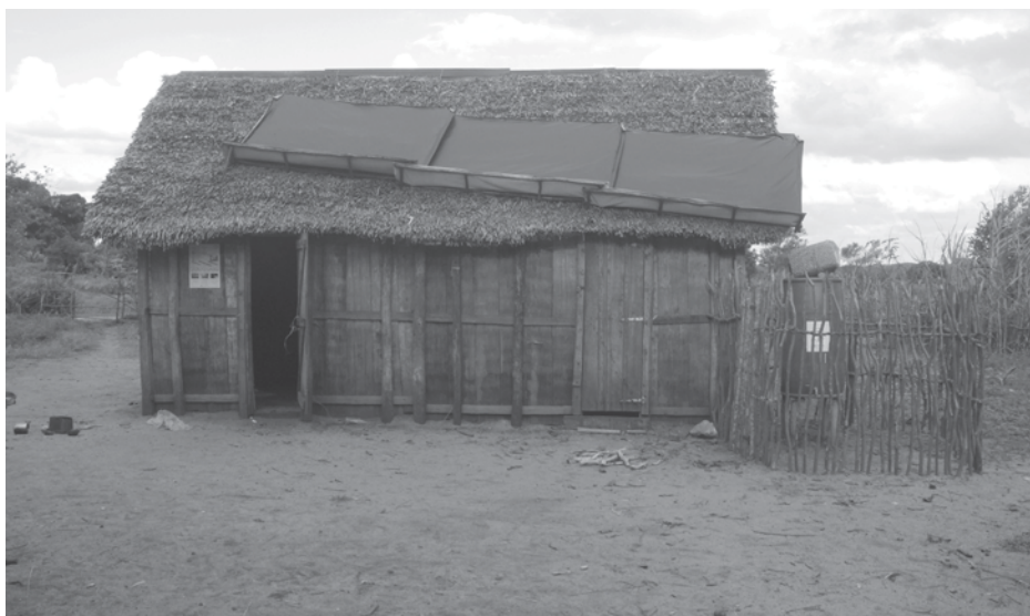
Photo 3 Innovative synthetic leather roofing panels retrofitted to a ravinala house
