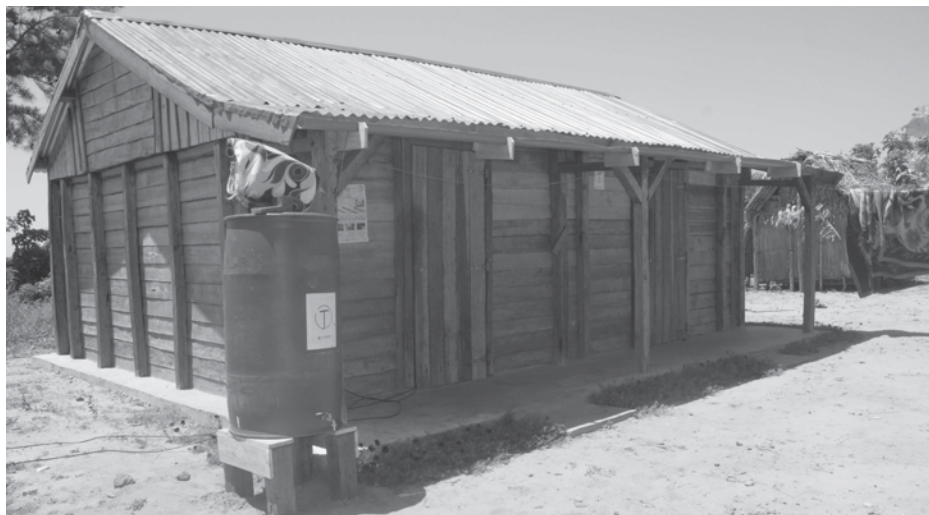
Photo 2 Conventional RWH system using metal roofing and plastic guttering
