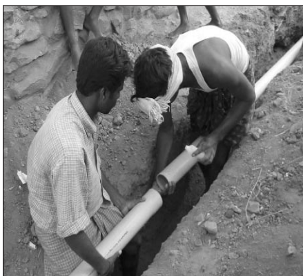
Installing a new pipeline in Battuvani Palli from the low-fluoride source
